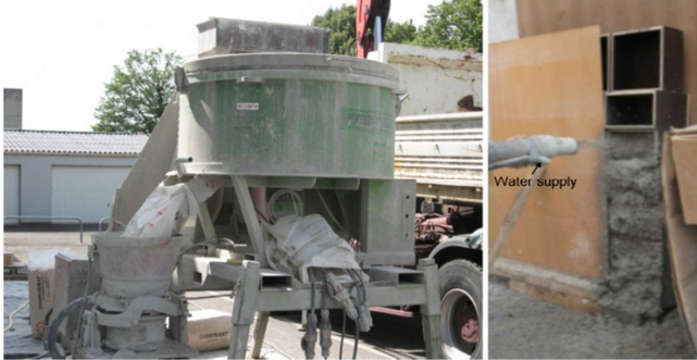
Figure 1. Spraying method (left : mixer, right : spraying hose)
